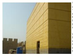
The crew sprayed between the 6-inch metal stud wall cavity of the 35-foot high gym. "We applied 2 inches for R-13," says Fitzgerald. "The gym is going to have sheetrock, and the auditorium and practice gym will have exposed block for the interior walls. In the auditorium we sprayed the block wall from the outside and from the inside they polished the CMU to make it look like it's prefinished stone."
